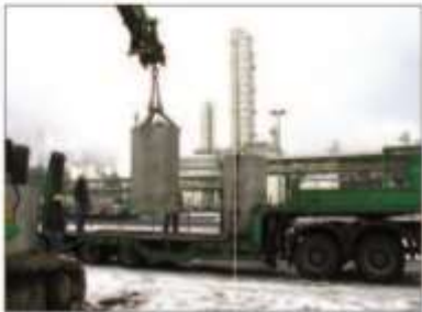
Loading and transport of the cat. soil monoliths
