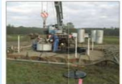
Insertion of the lysimeter into the station
