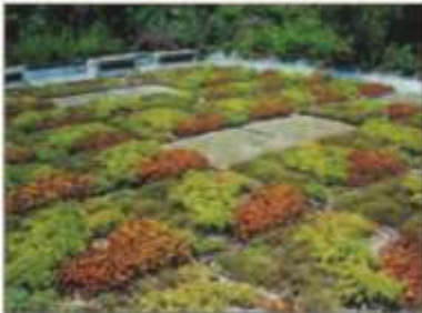
Lysimeters integrated in the green roof construction
