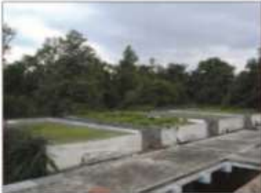
View over the test roofs with different vegetation systems
